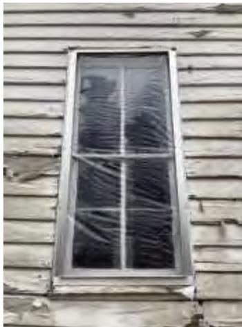
*Figure 5. Broken window covered in temporary plastic*
