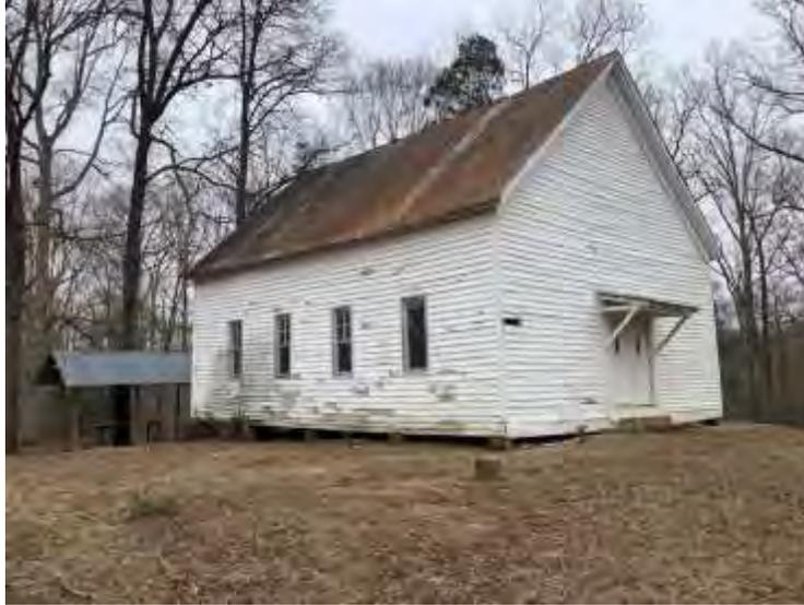
*Figure 4. Southwest corner of building showing peeling paint and missing weatherboard*
