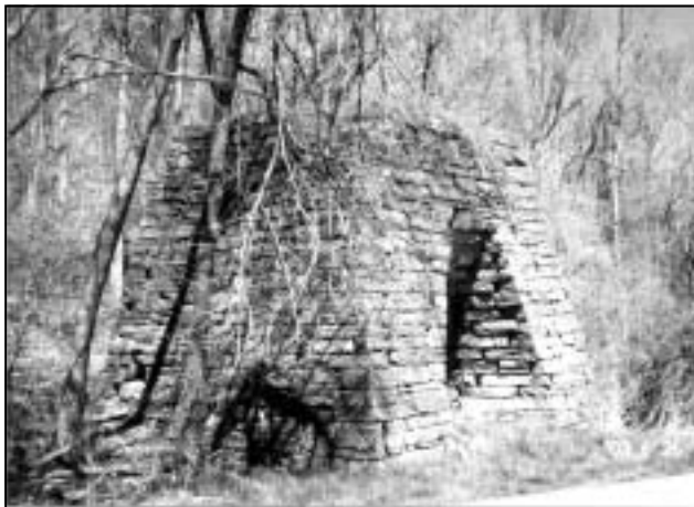
Remains of the Lee and Gould Furnace, built circa 1833-1835, in Hickman County.
